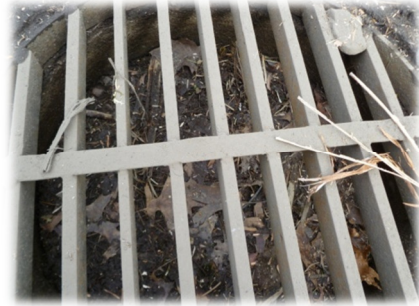
Figure 11 – Filled Catch Basin
