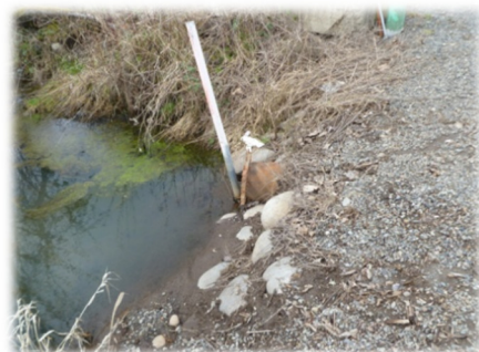
Figure 9 – Blocked Culvert
