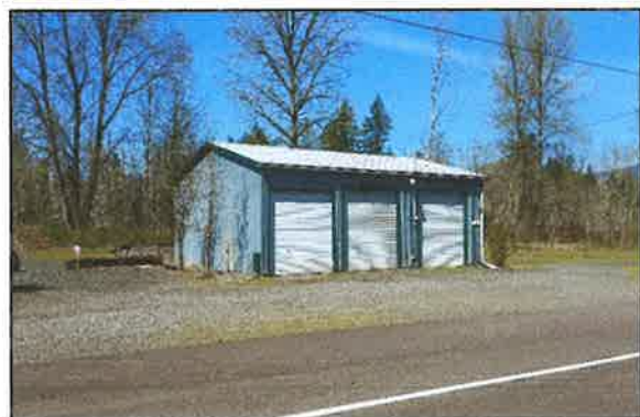
Shop, 725 N. 13 th Street
