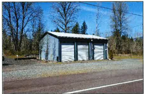
Shop, 725 N. 13 th Street
